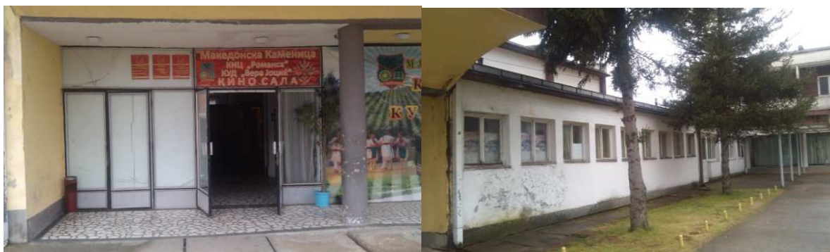
Figure 5 Details of the dilapidated and outdated exterior carpentry
